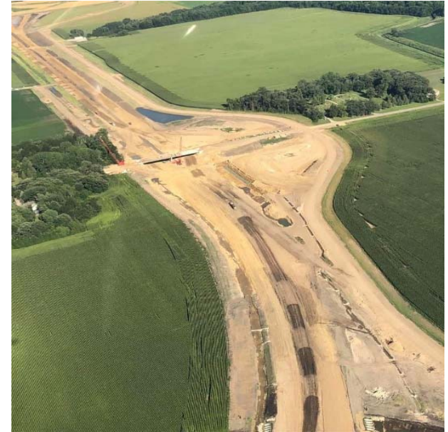
Dodge County CR 1 Overpass
