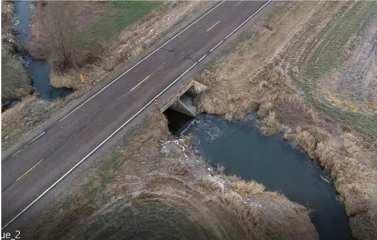
Photo 7: One of the two box culverts at the outlet is blocked by sediment.
