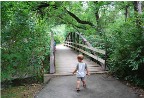
Trail bridges over ravines
