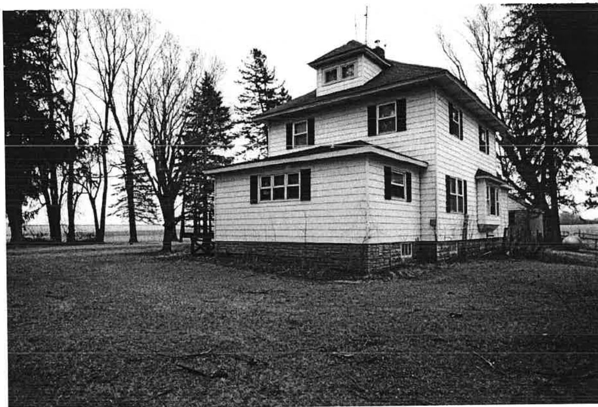
Photo #3: The NW corner of the existing home. This photo is taken facing the SE.
