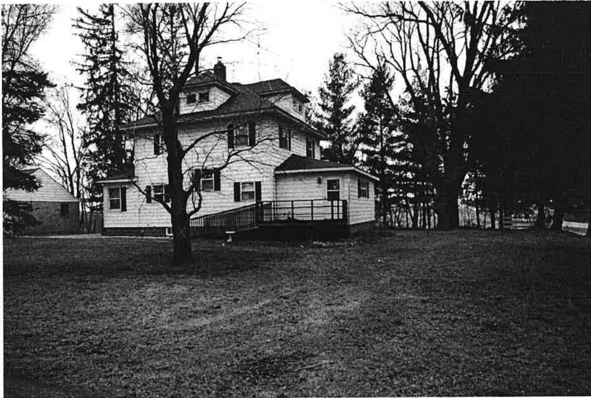
Photo #1: The North and East sides of the existing home. The photo is taken facing WSW from the existing driveway on the property. Country Road 12 is on the right-hand side of this photo.
