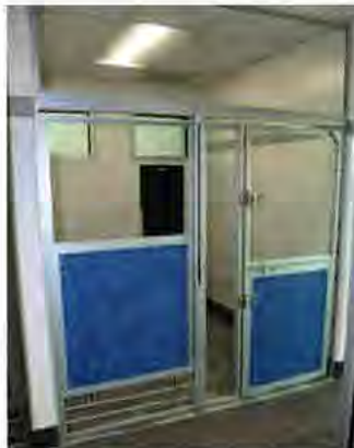
These tempered glass gates with privacy panels and clearstory upper front panels were custom designed for the Larimer County Humane Society, Ft. Collins, CO
