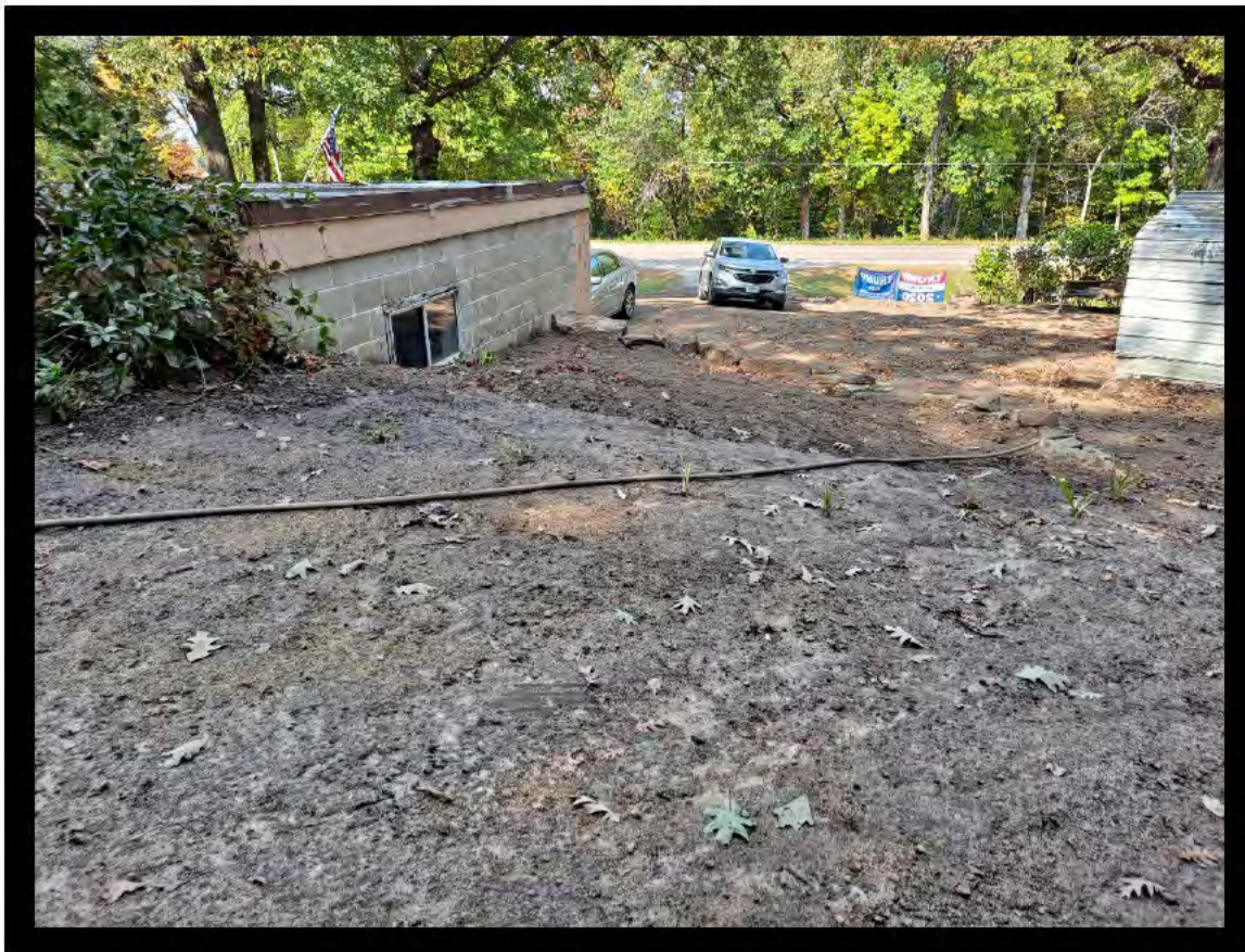
East side of garage standing on vehicle access to rear of dwelling – September 2020
