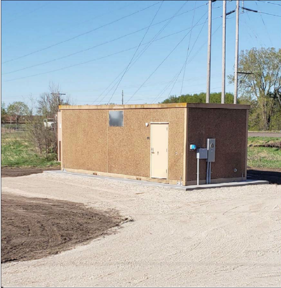
EXHIBIT A-1 Picture Depicting Tenant's Building Shelter is 8'x12'
