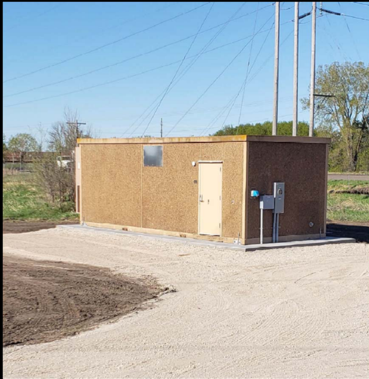
Typical Arvig Building Installation
