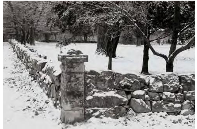
Winona Cottage Stone Wall Mortar Less Construction
